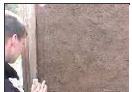
finitions stage Le Gabion (doc.Le Gabion)
