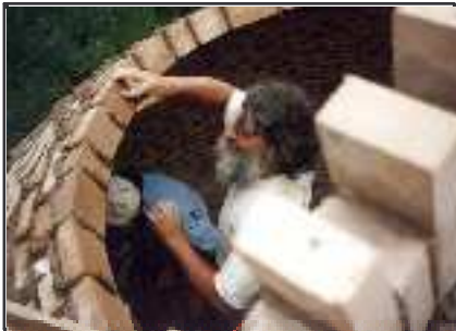
cule de four (doc.Le Gabion)
